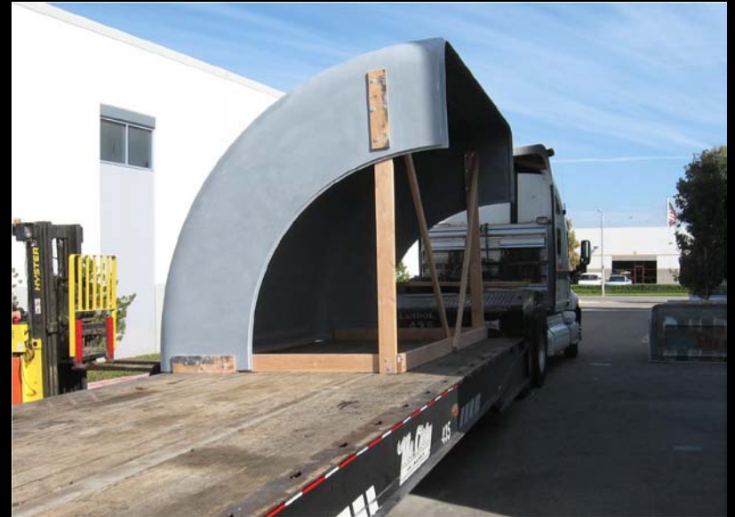
Transporting modular sections of cladding to site
