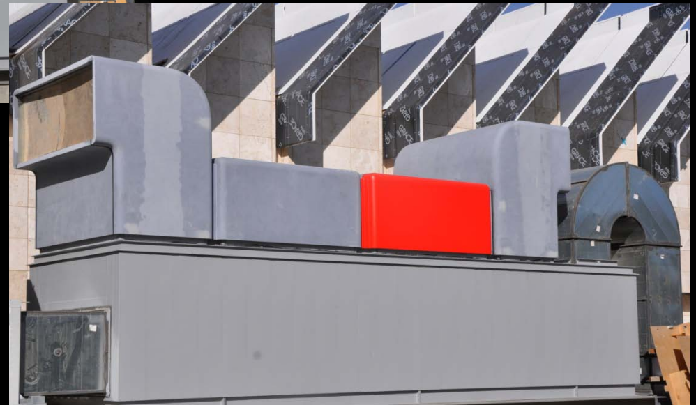
Los Angeles Construction Site
